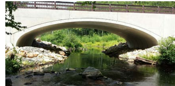
Undersized culverts limit water flow and are barriers to passage for fish and other wildlife (top and middle). Replacement structures are often much larger, provide capacity for larger water flows, and allow fish and wildlife to pass safely and freely (bottom).
